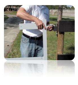
Drop the bearing into the barrel and place the smooth end of the J Bolt into the hinge barrel. Hold the gate frame the height off the ground you would like your gate to hang and hold the hinge plate against the post and mark its position.
